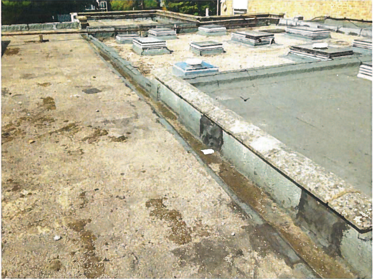
View from roof 5.jpg
